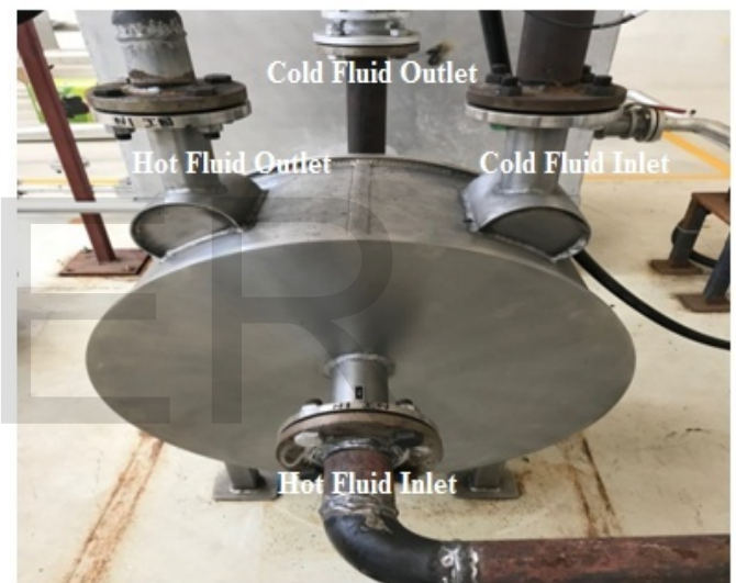
Fig. 8. Spiral plate heat exchanger setup
